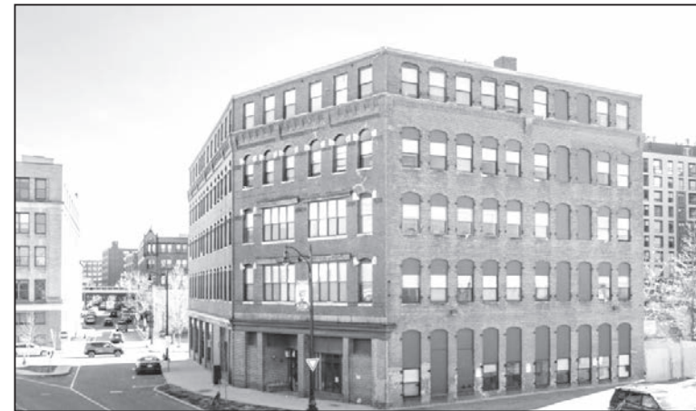
Olympia Square Apartments was recently acquired by POAH.
